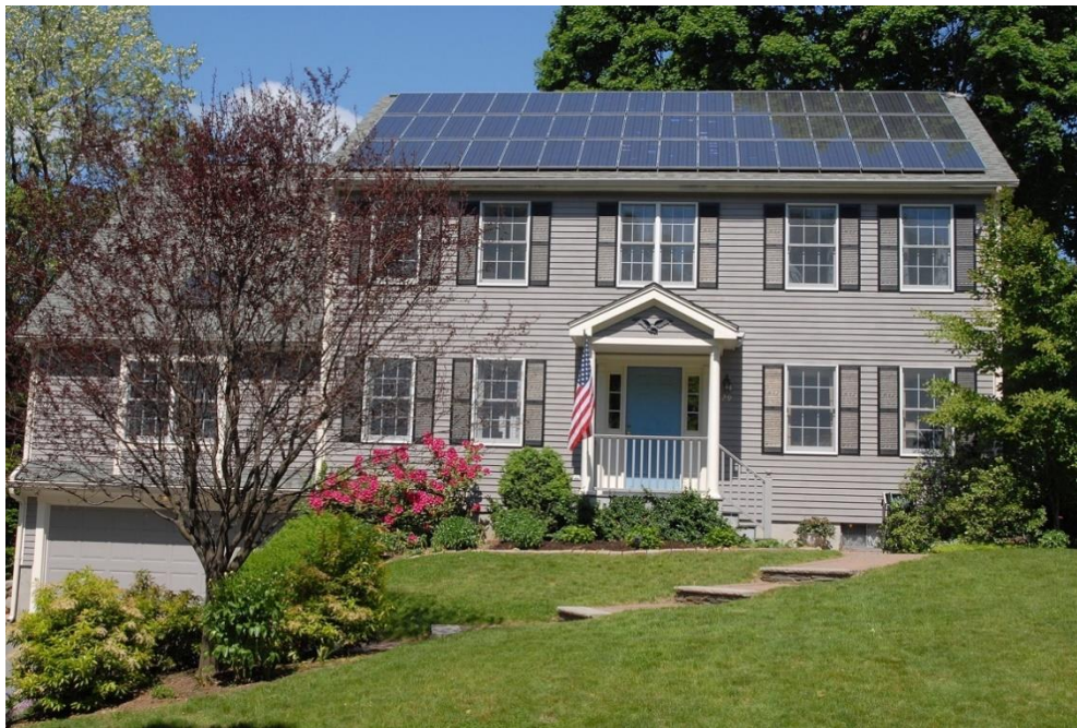
Solar rooftop system in Boston, Source: Wikimedia Commons
